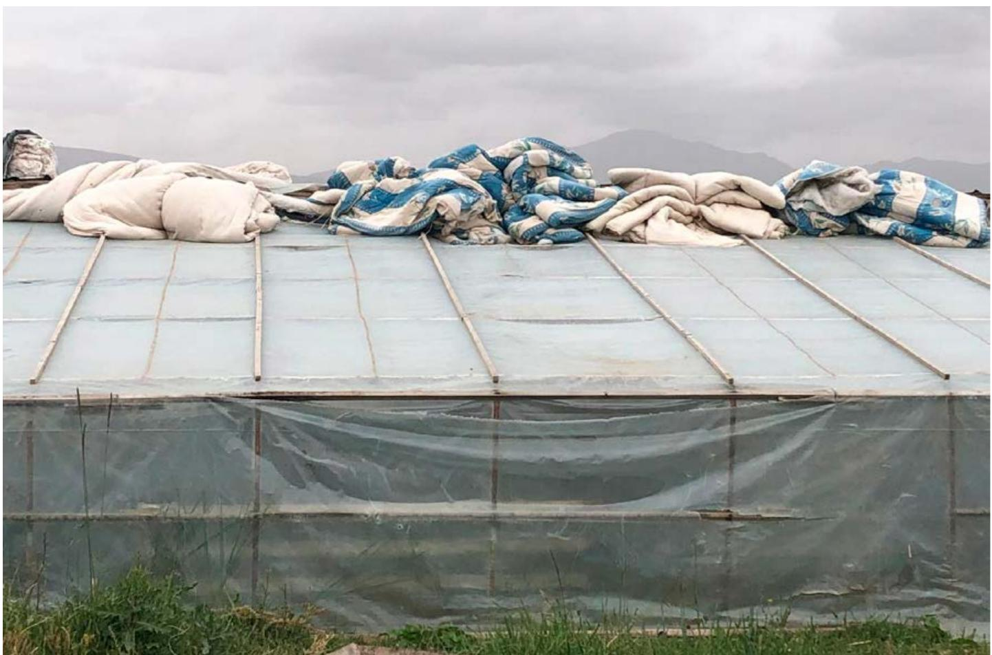
Figure 3: The pioneer greenhouse roof was lined with various kinds of textiles that were bound together and lying on the roof in order to provide the roof with an additional warm barrier against the cold. In Kyzyl-Tuu, the winter lasts between 5 and 8 months. Summers here tend to be colder and wetter than in other parts of Kyrgyzstan with an average temperature in July of 12 to 18°C.
